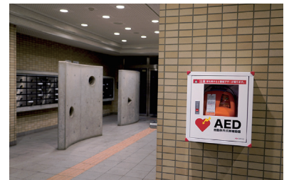
AED is installed in the entrance 1F
